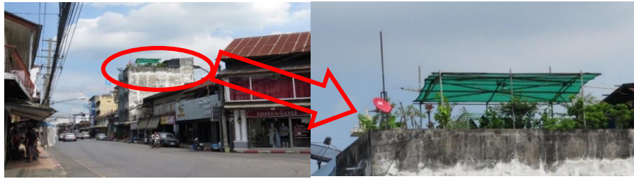
(a) Green roof
